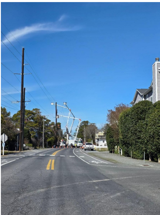
New Utility Poles Being
